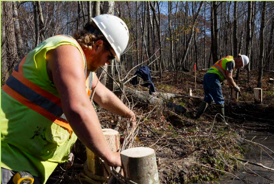
Employees weave sticks and tree branches while working on building a series of artificial beaver dams on Jim Hoffman's wooded property on Oct. 25, 2024, in Alma Center, Wis.
