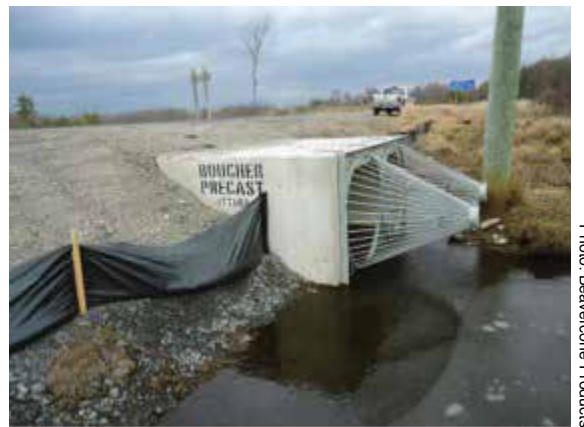
A Beavercone® installed on a culvert
