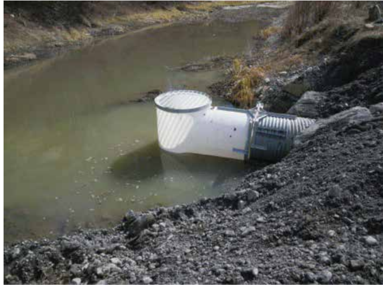
A Beaver Proof Add-On ® installed over a culvert
