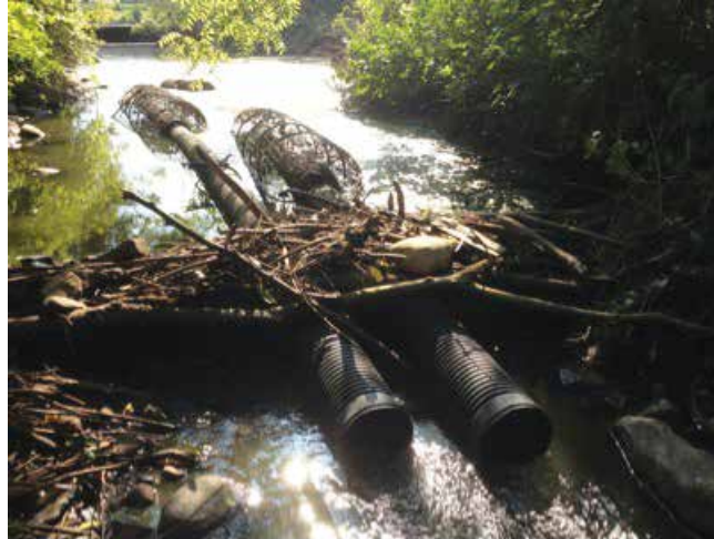
A Clemson Beaver Pond Leveler installed through a beaver dam
